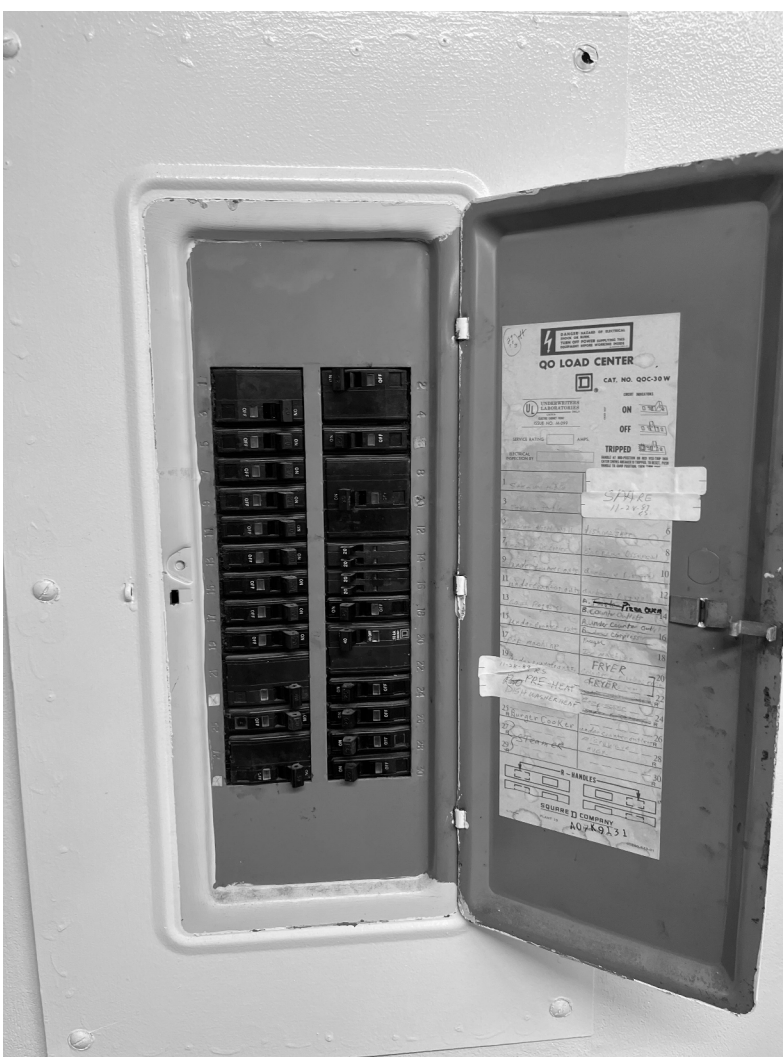
EXISTING PANEL B1 CIRCUITS TO BE REFEED FROM NEW PANEL B1 LOCATION. NOTE: PROVIDE TWO (2) SEPARATE BREAKERS IN LIEU OF TANDEM BREAKER.
