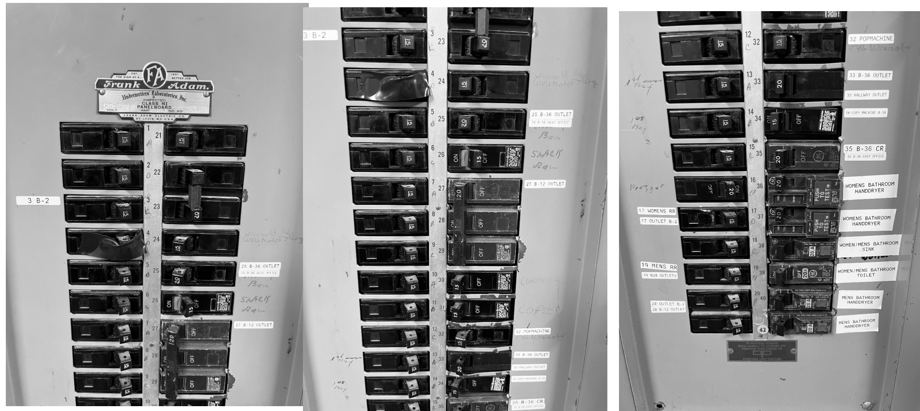
EXISTING PANEL L3 CIRCUITS TO BE REFEED FROM NEW PANEL L3 LOCATION.
