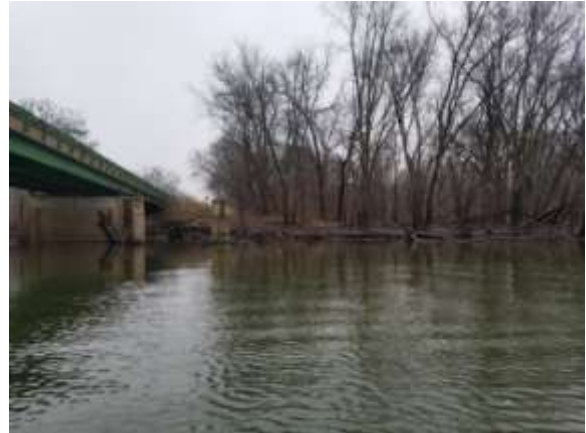
East end of the Cedar Wapsi (C-57) Bridge viewed from downstream _092443
