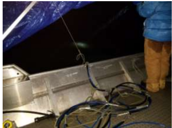
Watching diver at the Cedar Wapsi (C-57) Bridge _200538
