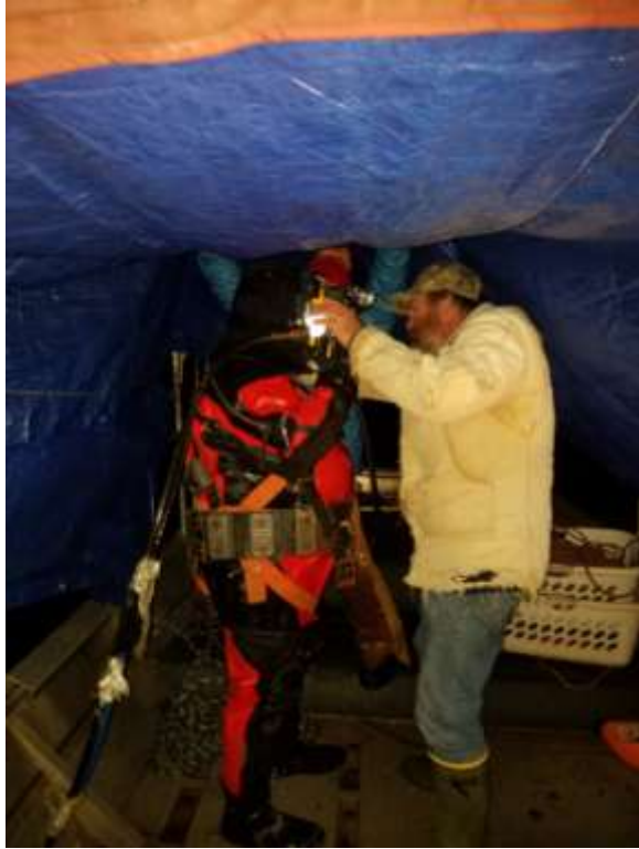
Diver suiting up at the Cedar Wapsi (C-57) Bridge _204437
