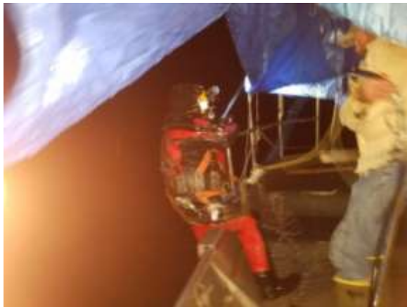
Diver entering water at the Cedar Wapsi (C-57) Bridge _200207
