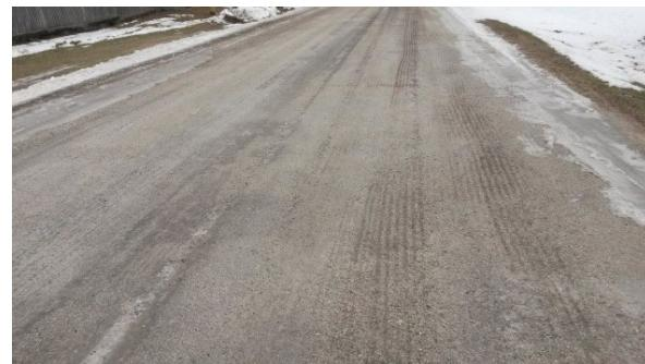
3. **Traffic Volumes:** if a road receives a high volume of traffic or has heavy agricultural use, it may not be cost effective to cover the roadway with a seal coat. Too many heavy loads can damage a seal coat. Particularly during the spring thaw, as was explained above.
